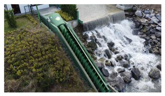
YEO, one of Türkiye's leading engineering and technology companies, in cooperation with its subsidiary Mikrohes, offers a renewable energy system that is completely environmentally friendly. With the Archimedes Screw turbine, energy can be produced from a stream of water with low flow and head. The system, which is nature and fish friendly, is shown as the technology of the future in this field as a zero-carbon method that does not disturb the balance of the region...
